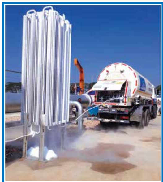
Nitrogen gas charging activities at Shalimpur point of Chattogram-Feni-Bakhrabad Pipeline
