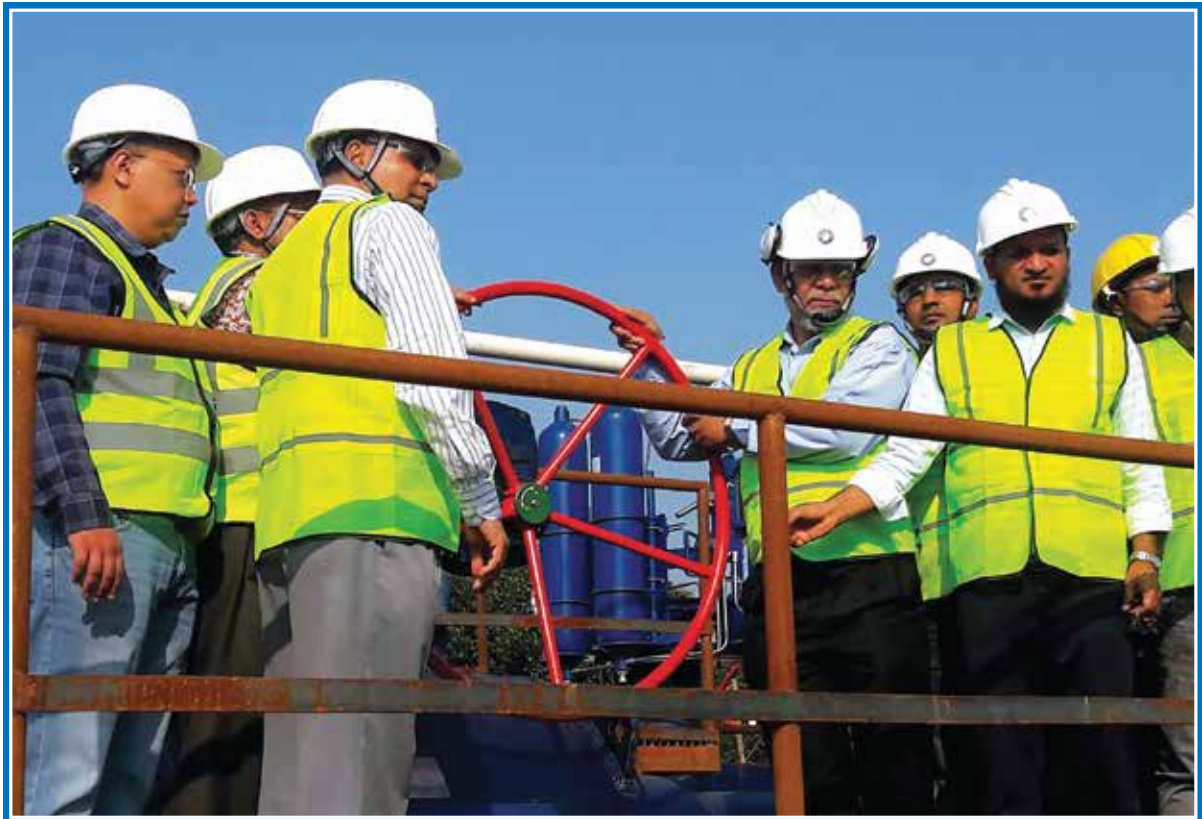
Pipeline commissioning of 36" X 181 k.m. pipeline under C-F-B project
