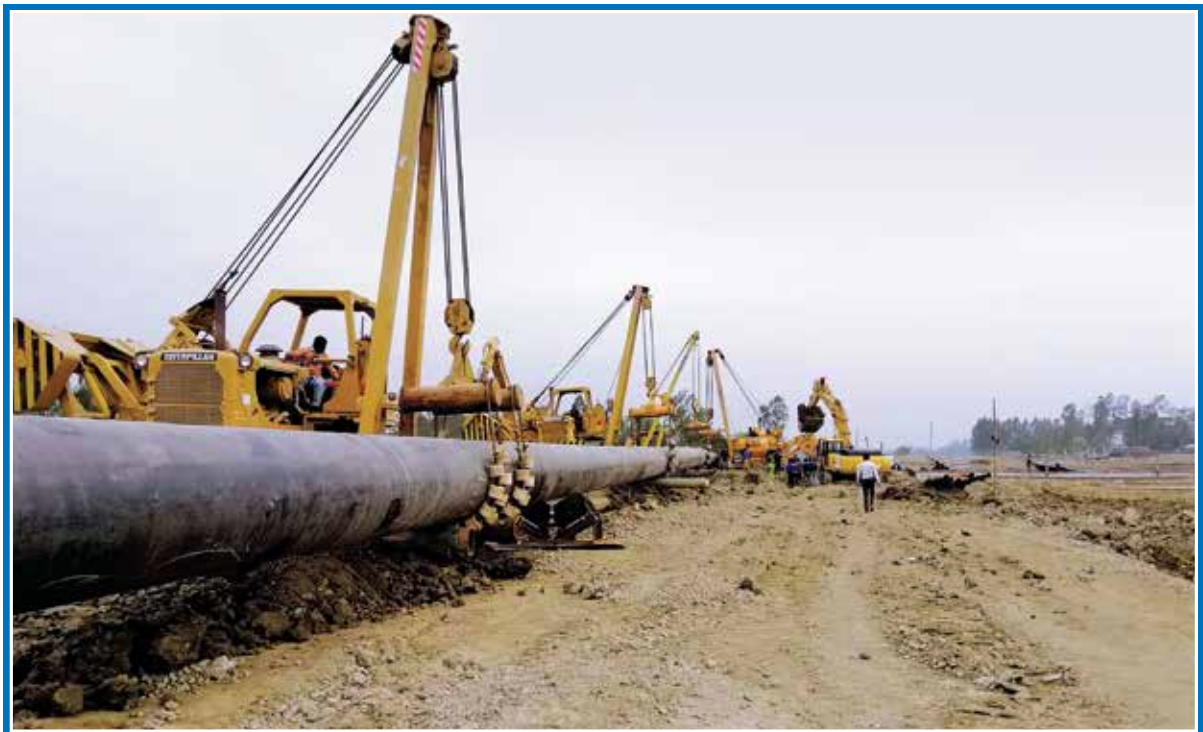
River crossing activities by HDD method under Moheshkhali-Anwara parallel project
