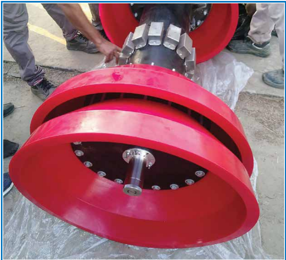
On stream pigging of 30" X 84 k.m. Hatikumrul-Bheramara pipeline
